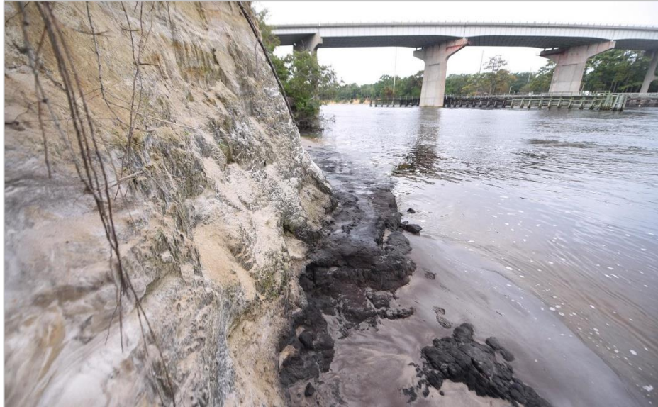
Figure A7.3 - Southern bank, looking west. The old swing bridge was in the background, in way of the power poles. Some shoreline areas have what appears to be consolidated substrate, which would tend to reduce the rate of erosion. Compare this to Figure A7.3.
