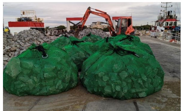
Figure 4: Medium rock bag prior to being placed in the water
