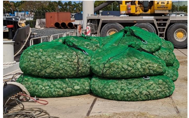
Figure 3: Small rock bag shape when stacked and filled to approximately 1.8 t
