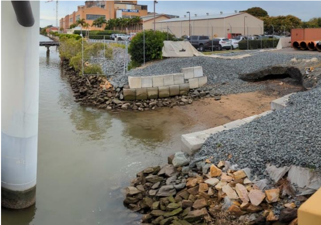
Figure 5: Original condition of test area
